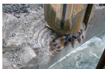
Drilling the existing RC Revetment
