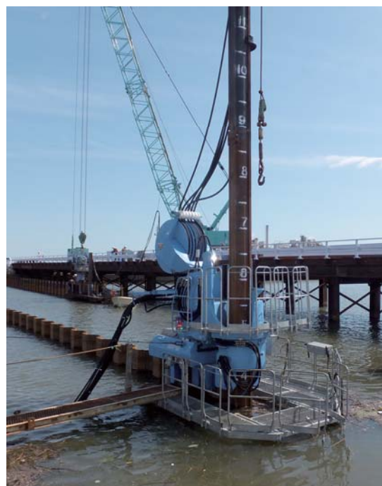
Drilling the existing RC Revetment
