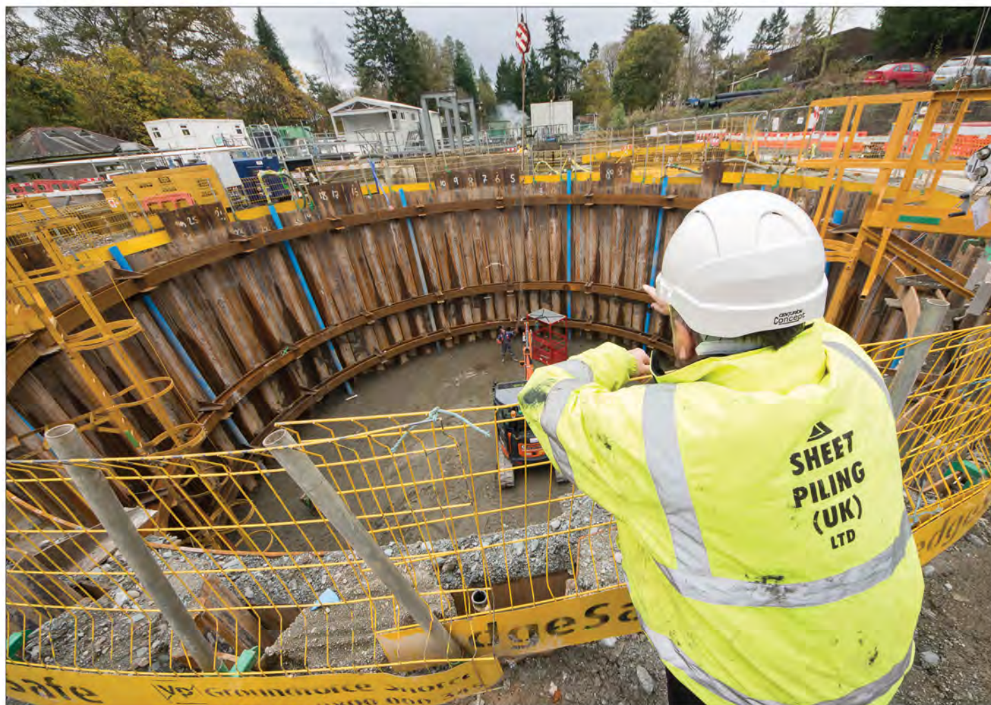
Photograph Above. Here's one we prepared earlier: A sheet piled shaft
