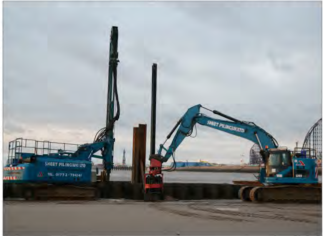
Photograph Above. SPUK undertaking sheet piling in Blackpool
