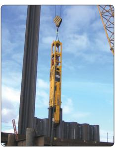
CX85, Crane suspended and fitted with legs and inserts for driving sheet piles
