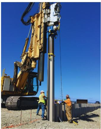
Driving any sheet piling material to significant depths is a challenging task. PileClaw® Installation Equipment, from CMI, offers a range of solutions developed to increase the likelihood of driving the company's ShoreGuard® and UltraComposite™ synthetic sheet piling to desired depths. PileClaw Installation Equipment's proprietary technology offers 20 years of documented performance. And,
